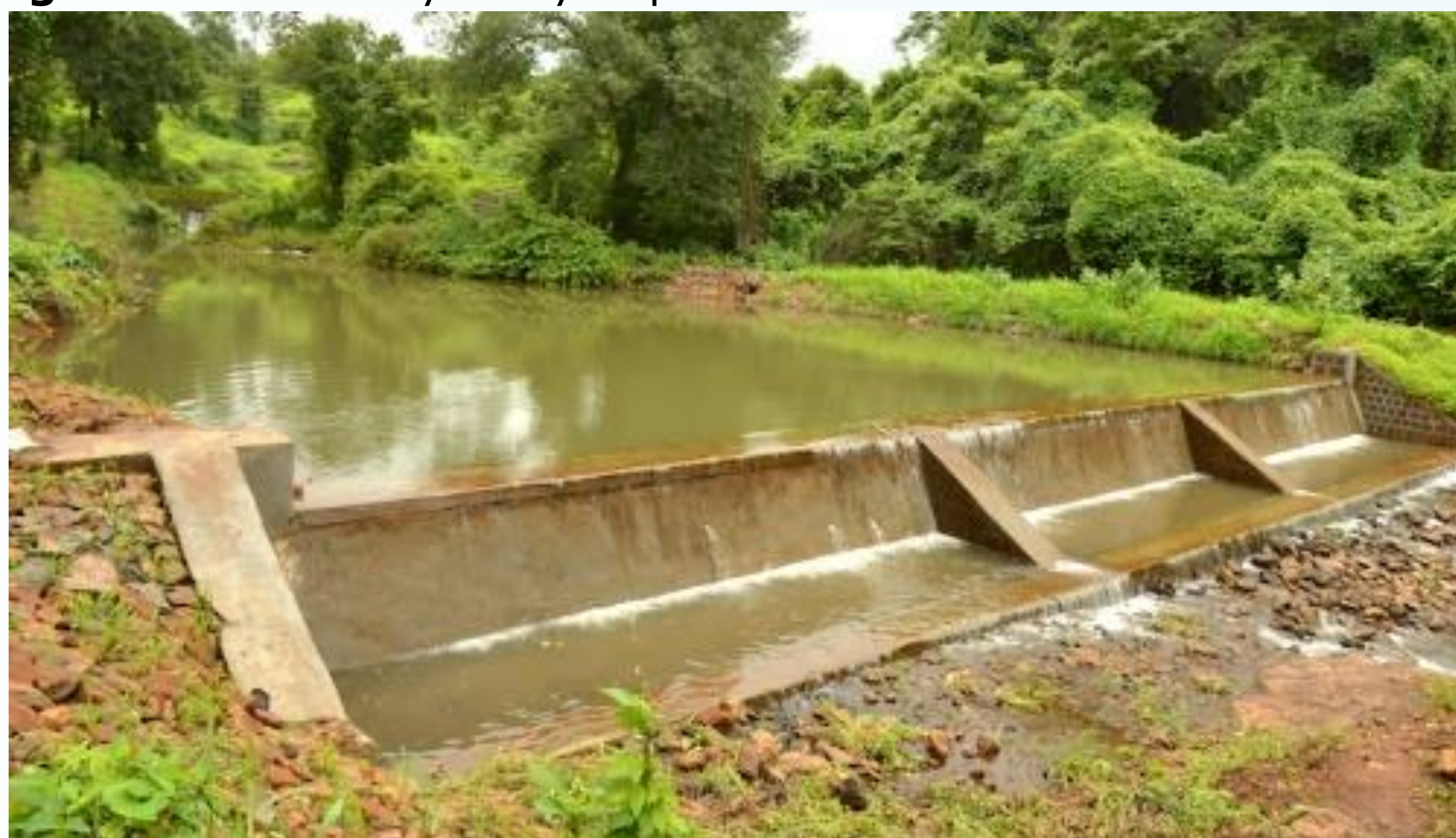
Photo 1. Constructed dam to address water scarcity
